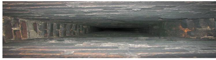
The interior of this chimney has heavy creosote deposits and if not removed, a blockage or chimney fire will occur.
